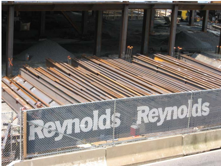
Steel Staging on Market Street
